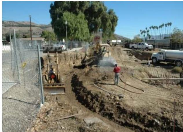
Below: Wetting down the dusty dry earth is essential to dust control and proper compaction of the soil. A large water tanker (out of sight left) provides the needed water.
