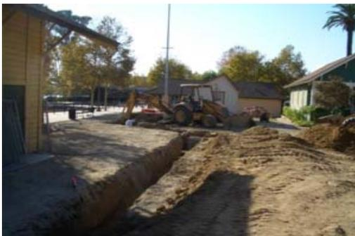
Above: We see construction equipment compacting the hoop rail foundation and digging the access pit for the table. Right: Accuracy in turntable construction is critical. Tolerances are very tight between the center pivot and the hoop rail. Here we see construction workers taking additional depth readings for the pit perimeter foundation.
