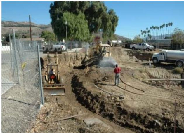
Above: We see construction equipment compacting the hoop rail foundation and digging the access pit for the table. Right: Accuracy in turntable construction is critical. Tolerances are very tight between the center pivot and the hoop rail. Here we see construction workers taking additional depth readings for the pit perimeter foundation.
