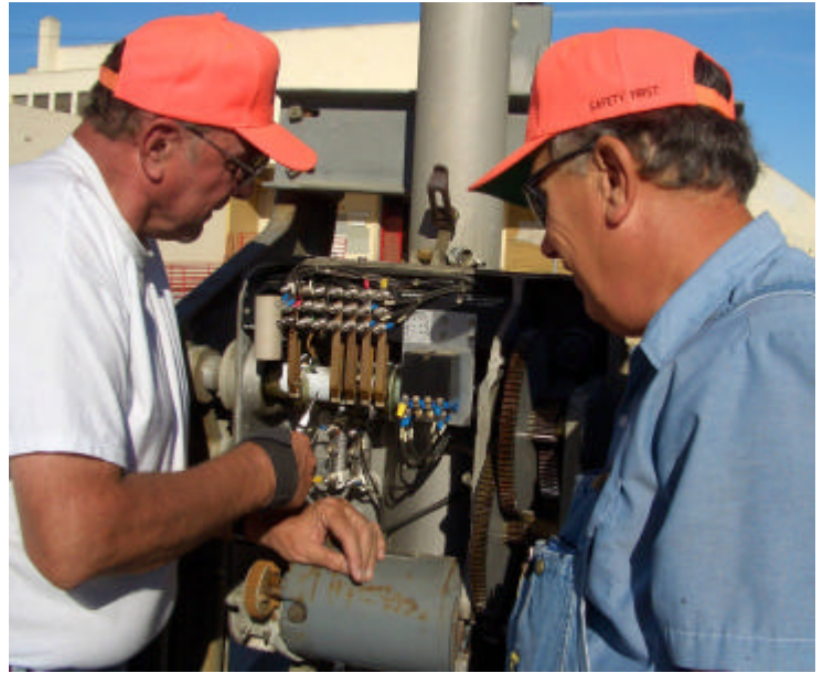
SCRVRHS members Mike Morgan (L) and Greg Schmidt (R) tune up one of many Fillmore & Western crossing arms in preparation for the heavy Christmas Tree and North Pole Express train traffic in December. Come visit Fillmore and take a F&W train ride!
